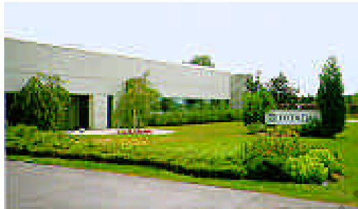
Hitachi Kokusai Electric America, Ltd. Headquarters, Woodbury, NY
